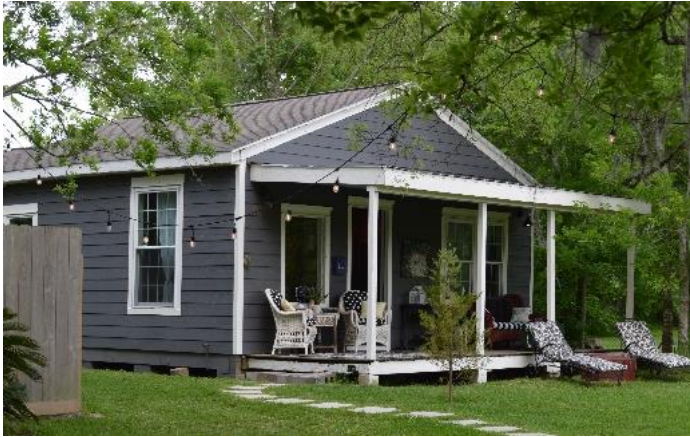
Guest house built in 1937 from wood salvaged from World War I barracks at abandoned Ellington Field LCDR Joyce Zongrone USN (Ret.)
