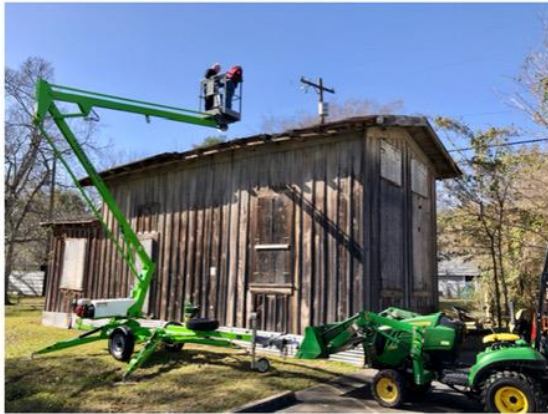
Richard Lewis & friend placing tarp on roof.
